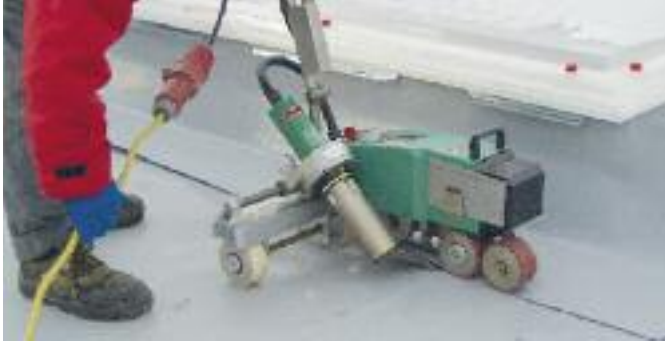
Due to its slim line design, welding is possible even in close to edge spaces.
