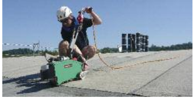
Flameless modified bitumen welding with the BITUMAT B2.
