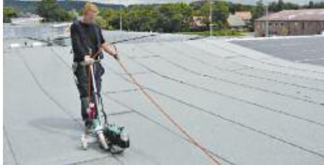
Easy unit guidance and clean working with the BITUMAT B2.
